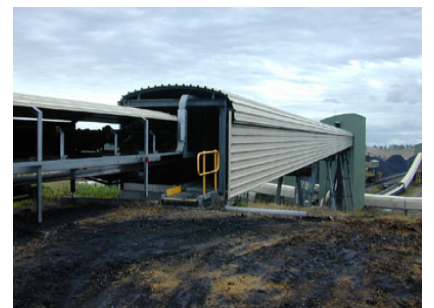
Entering crushing station
