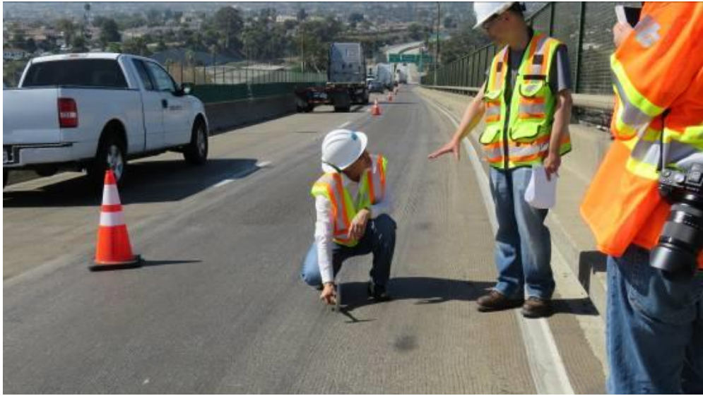
Vincent Thomas Bridge 橋梁檢測作業情形
