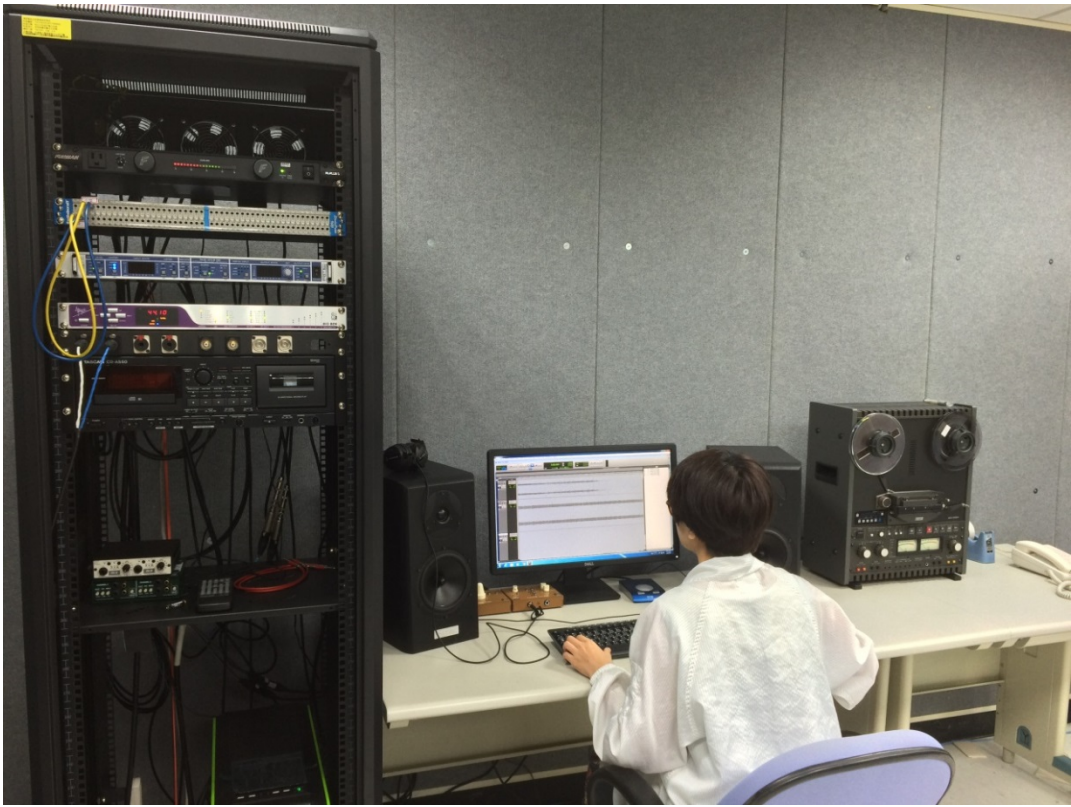
Figure 7 Multimedia Archives Conversion & Repair Area (2)
