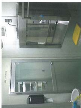
Get changed in the preparation room and pass through the air shower to enter the laboratory.
