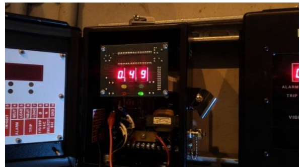
圖 30 vibration sensor receiver 顯示正常
