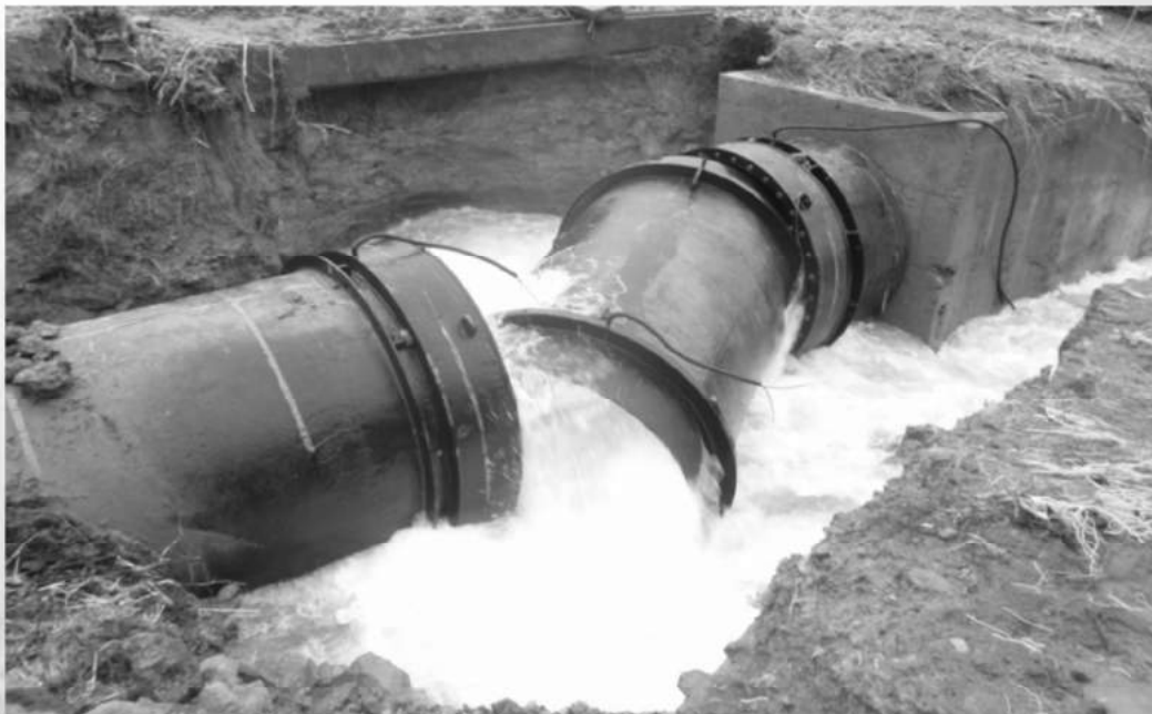
φ2400mm Pipe (Flexible Joint), Sennan-Senen Regional Waterworks by Miyagi Prefectural Government
