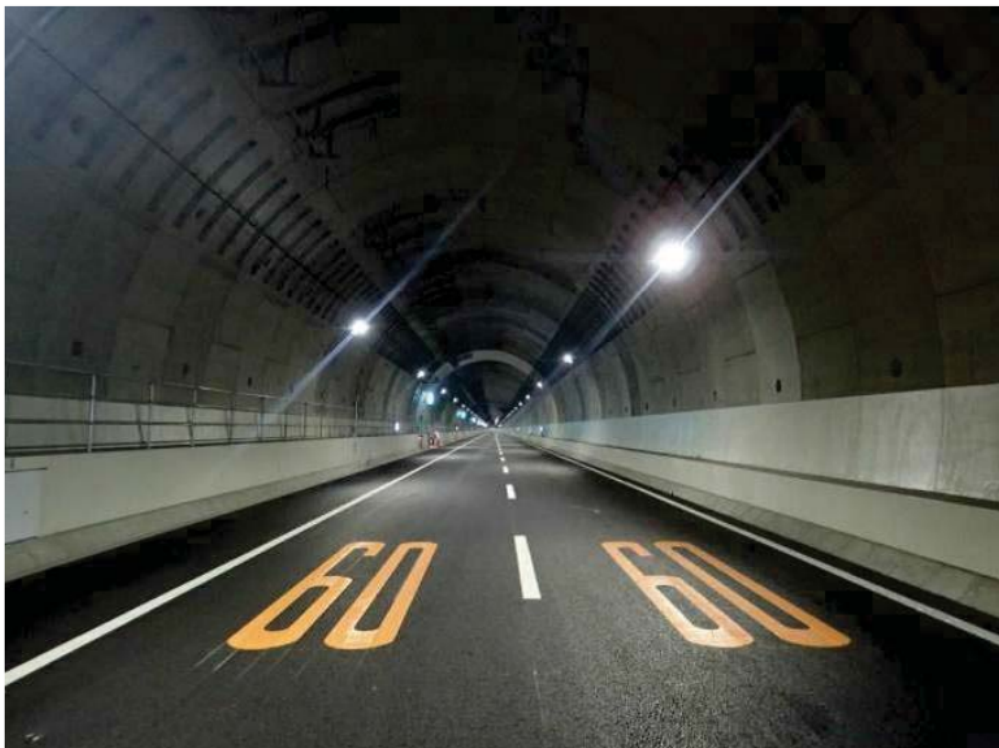
The Construction of Yamate Tunnel on the Central Circular Route by Metropolitan Expressway Co., Ltd
