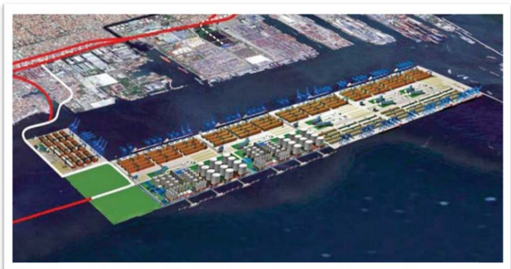
Development of North Kalibaru Container Terminal Phase I Port of Tanjung Priok by New Priok Port Project I PT. PP (Persero) Tbk.
