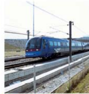
Ground Transport 陸路運輸
