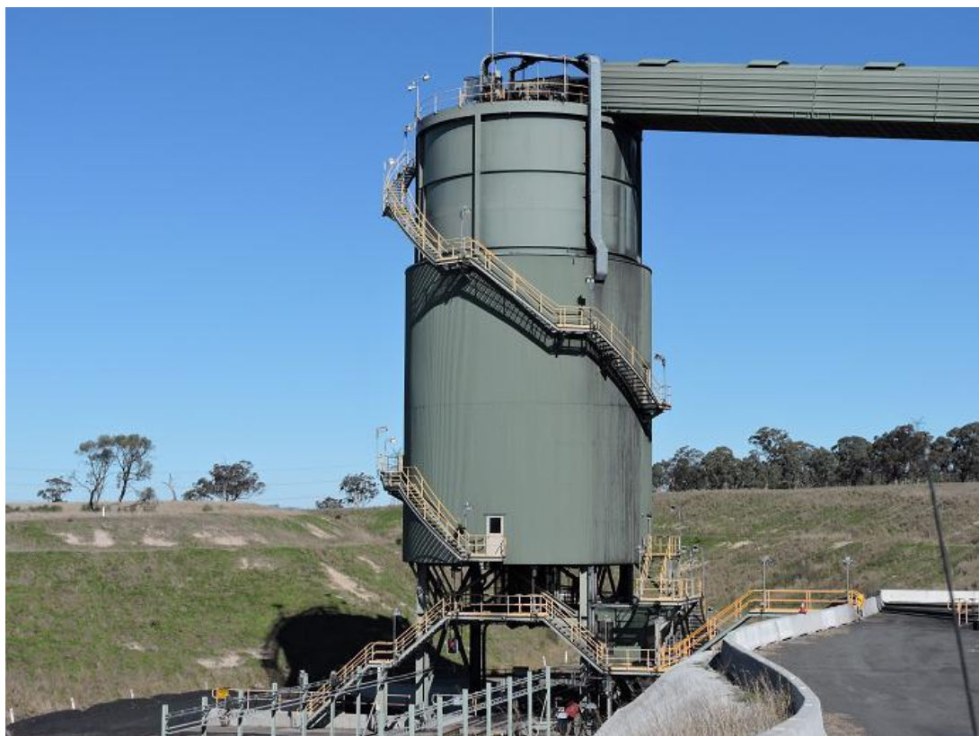
圖29 Mangoola礦區火車裝運站(Train Load Out)
