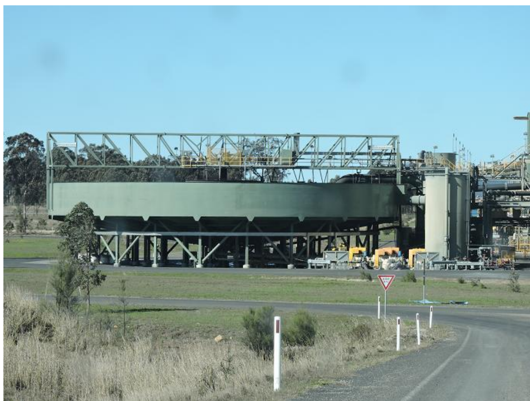
圖18 Mangoola礦區CHPP之Thickener
