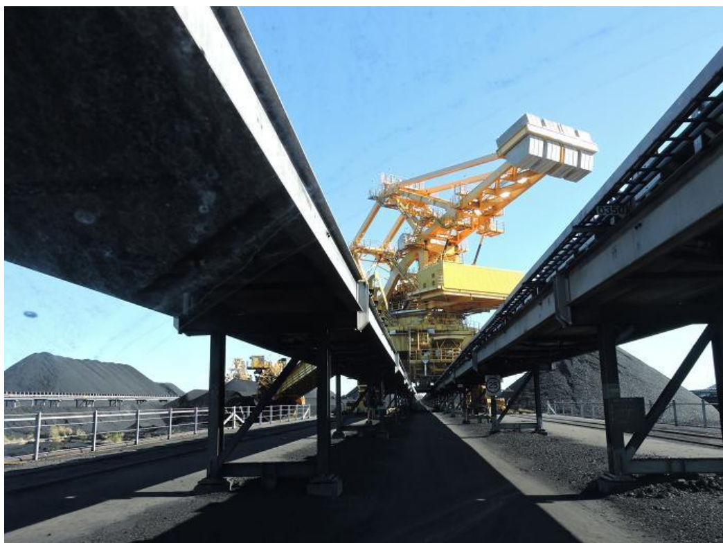
圖40 PWCS斗輪式堆/取煤機(Bucket Wheel Stacker/Reclaimer)
