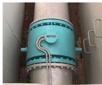
Electromagnetic meter (Check every month)
