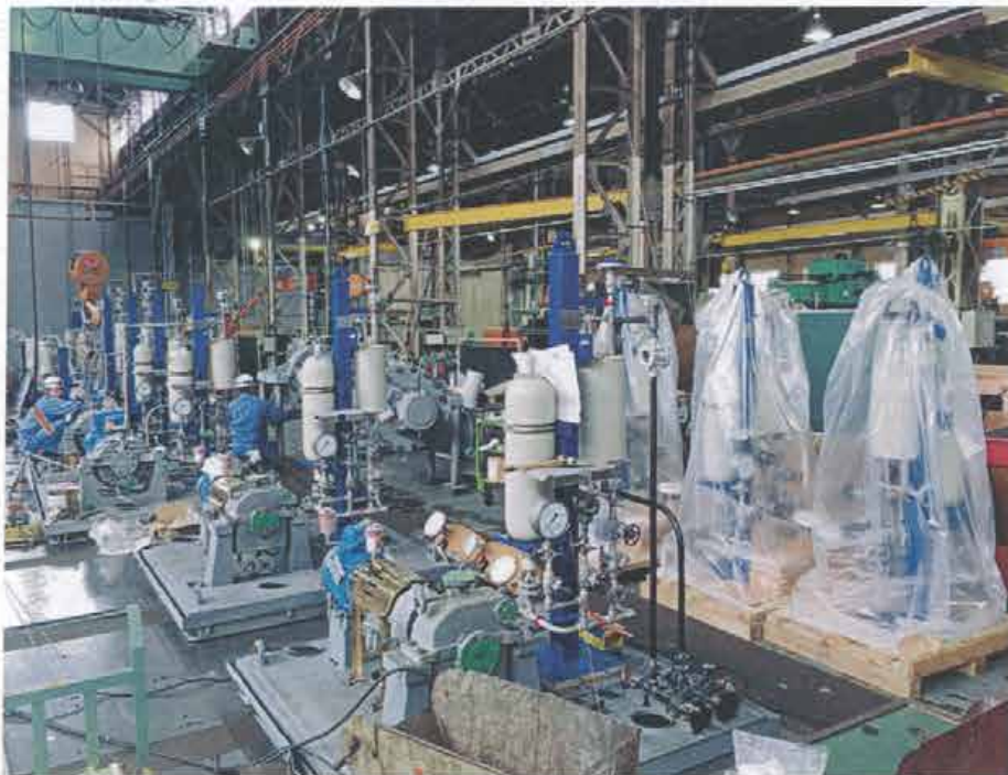
Pipping and Alignment
