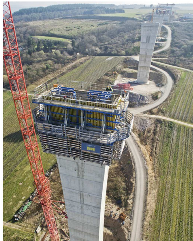
View of the automatic climbing form work Image: Brückner
