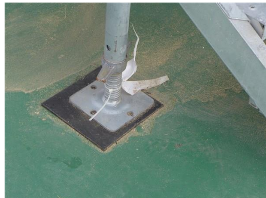
租賃組裝式看台角柱加設橡膠墊
