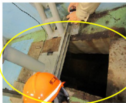
Opening of the traveling screen's manhole (El. 6.6 meter)
