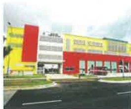
Banyan Fire Station
