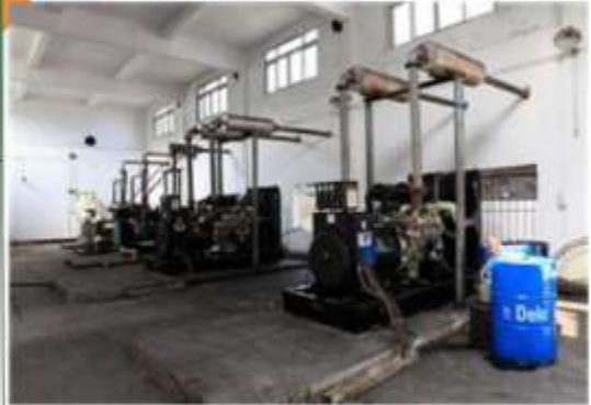
1000kW diesel generation units
