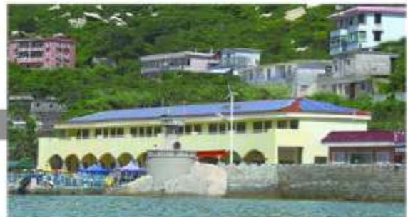
PV system in multifunctional building
