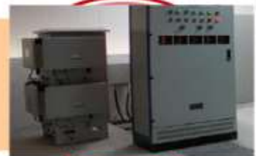
Grid-connected inverter for wind turbine
