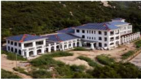
Sub-microgrid in culture center
