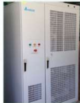
250 kW bi-directional inverter
