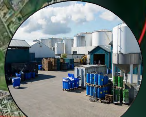
Transfer station for hazardous waste
