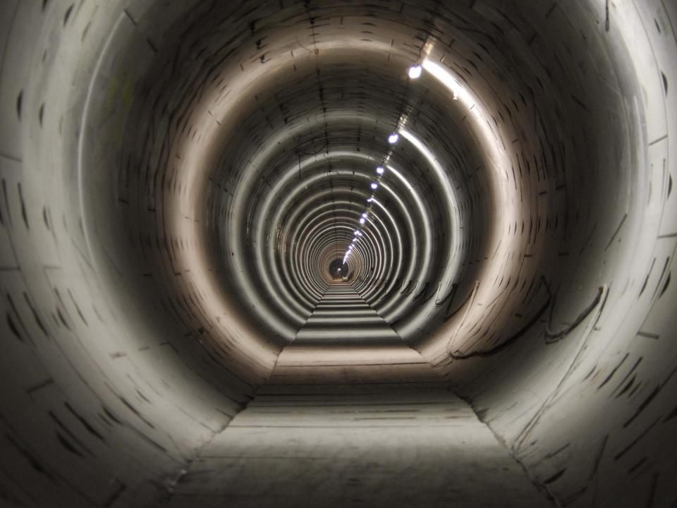
Inner lining with membrane in skaft and og NATM tunnel
