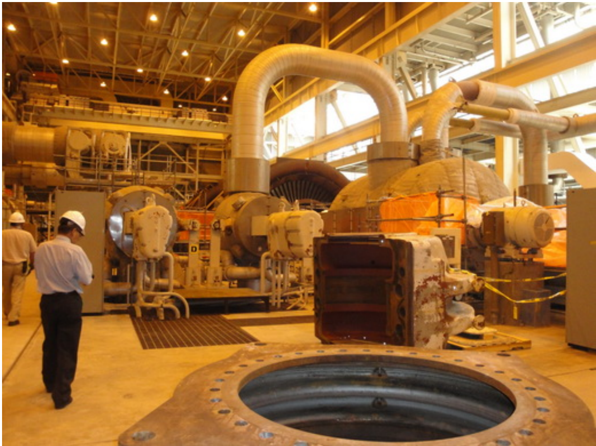
汽機軸承蓋拆開後已不回裝
