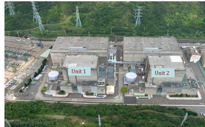
Bird Eye View of Power Block Chinshan NPP
