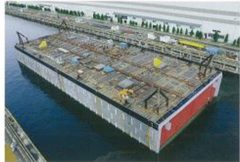
沈没函 Immersed tunnel
