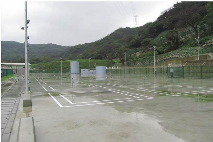
Independent Spent Fuel Storage Installation (Phase I) 11
