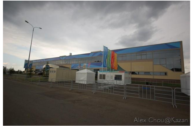
2-1b. “Kazan” Equestrian Complex Indoor Hall 外觀
