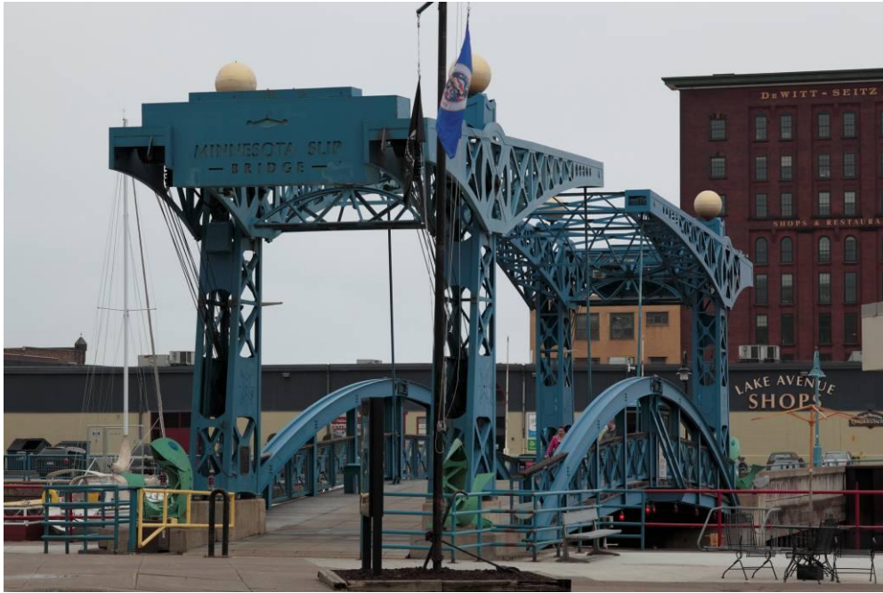
圖 211.9 Minnesota Slip Drawbridge
