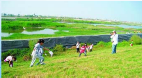
Rive bank restoration near Erren River (2006)
