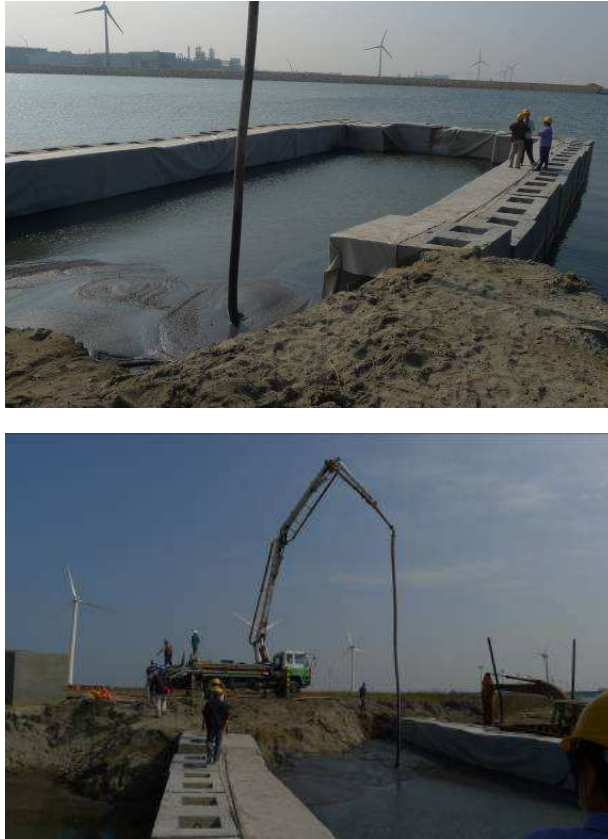
Figure 11 Photos of construction site
