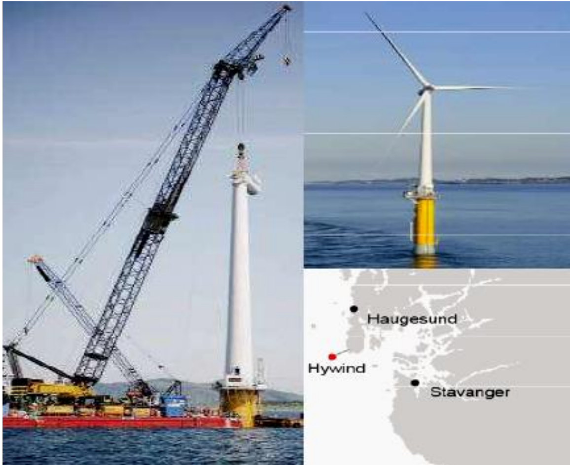
圖六：The World's first floating turbine In 2009 Siemens installed the first turbine in Norway at a water depth of about 220 meters
