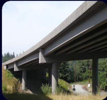
Example Bents Used with Prestressed Concrete Girders
