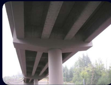
Example Bents Used with Prestressed Concrete Girders
