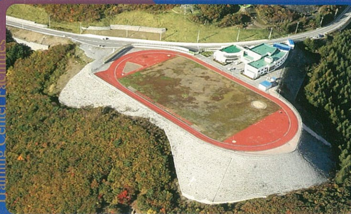
TAEBAEK Training Center Facilities
