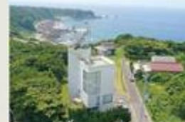
Research building with wind tower (Shionomisaki Wind Effect Laboratory)
