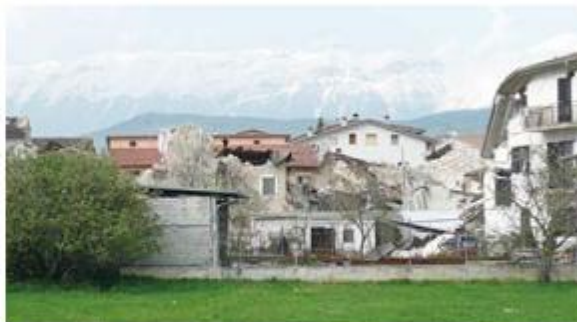
Severe building damage in the town of Onna from the 2009 L'Aquila, Italy earthquake
