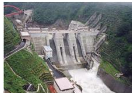
Sediment flushing of Unazuki dam, Kurobe River
