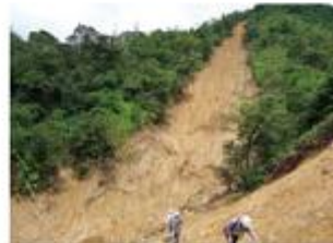
Shallow landslide in the granitic area of Hofu city by a heavy rain storm on 21 July, 2009
