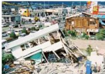
Collapsed houses in Nobeoka city induced by tornado on 19th September 2006
