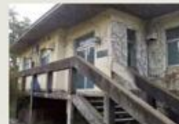
Main building (Ogata Wave Observatory)
