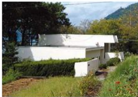
Tokushima Landslide Observatory
