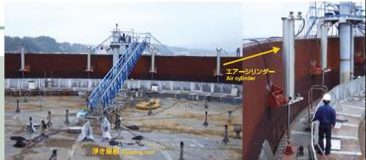
実際の浮き屋根式石油タンクを用いた浮き屋根の揺動実験 Experiment to assess the behavior of a floating roof in liquid sloshing in an actual oil tank
