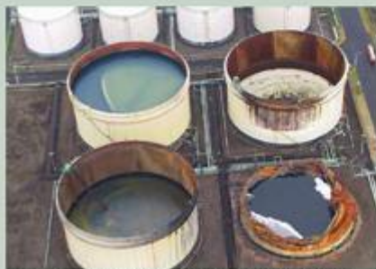
2003年十勝沖地震で「浮き屋根」が沈没した苫小牧の石油タンク Tomakomai oil tanks in which the floating roofs sunk during the 2003 Tokachi-oki earthquake
