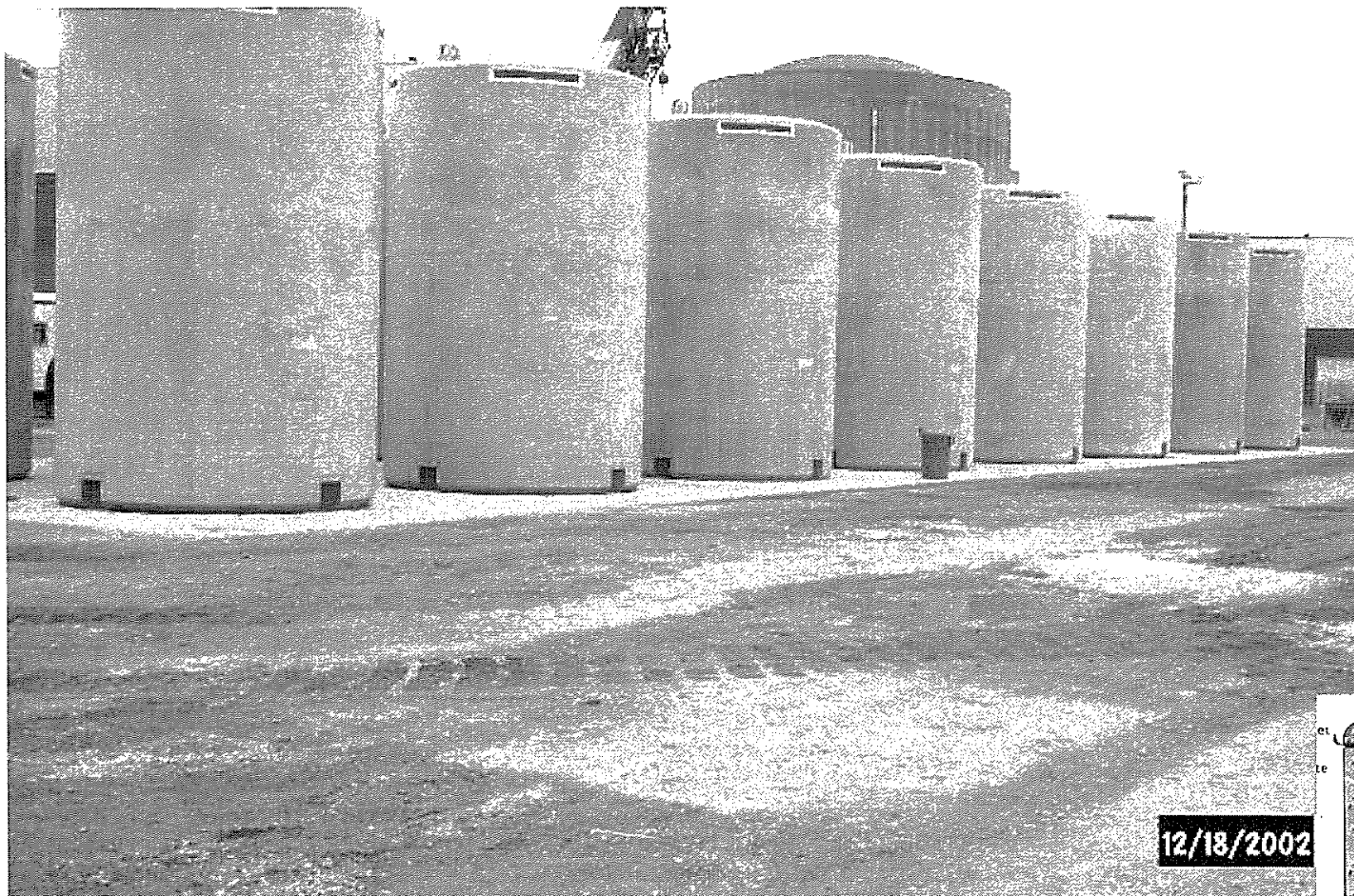
VCC After Construction
