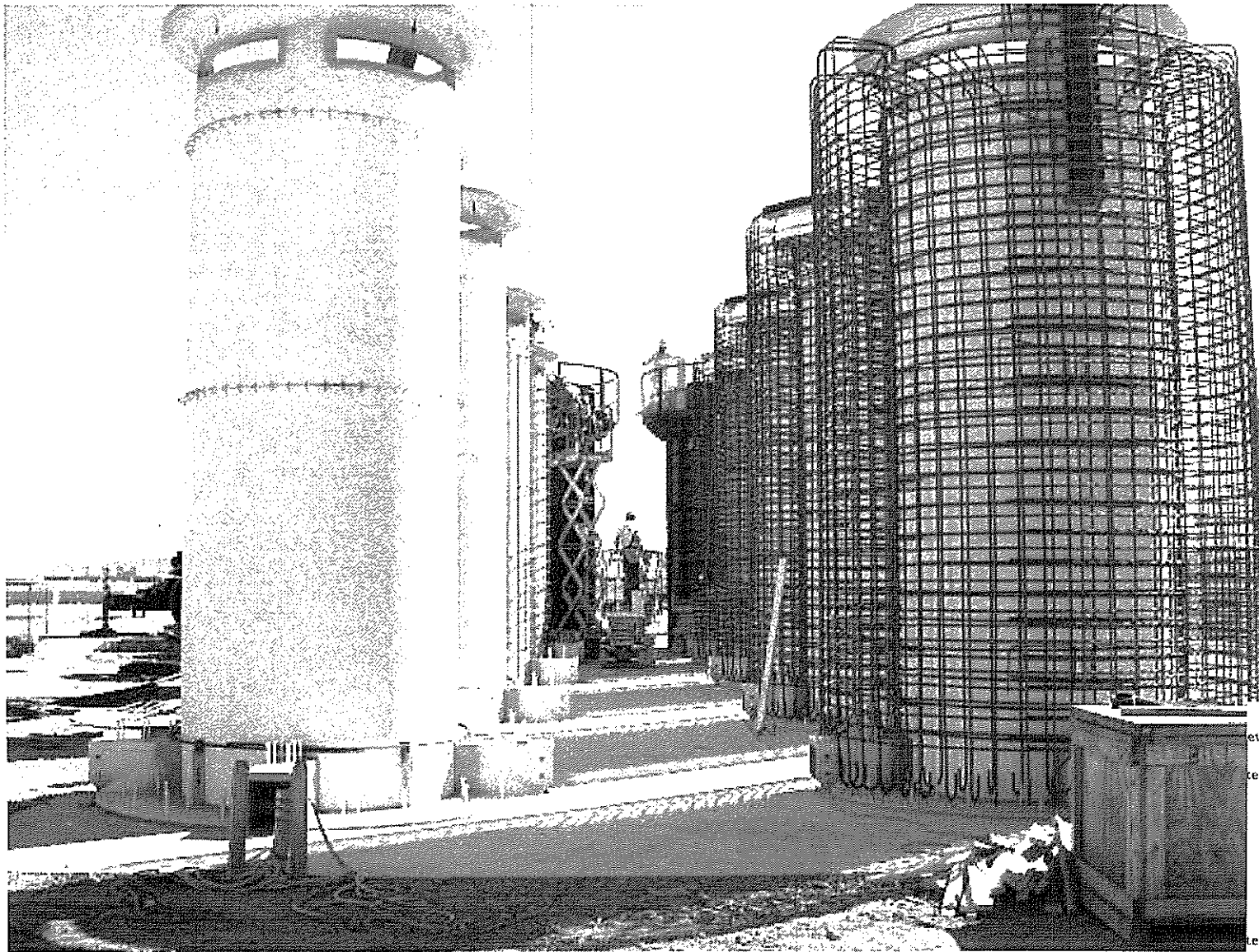
VCC Liners and rebar
