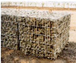
part of the gabion wall
