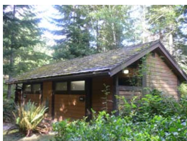
Lake Crescent 區步道旁公廁
