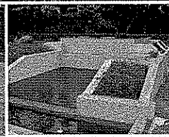
A 1,100-ton rainwater collection system for irrigation to conserve water resources 11,600 tons annually and to increase stormwater detention up to 85 minutes.
