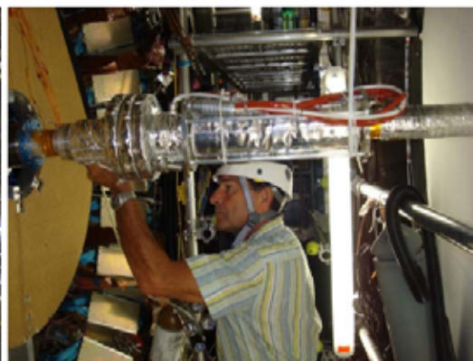
Connection of the ID section to the LAr EC beam pipe section
