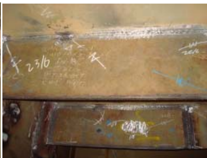
No.4S Steel Work
