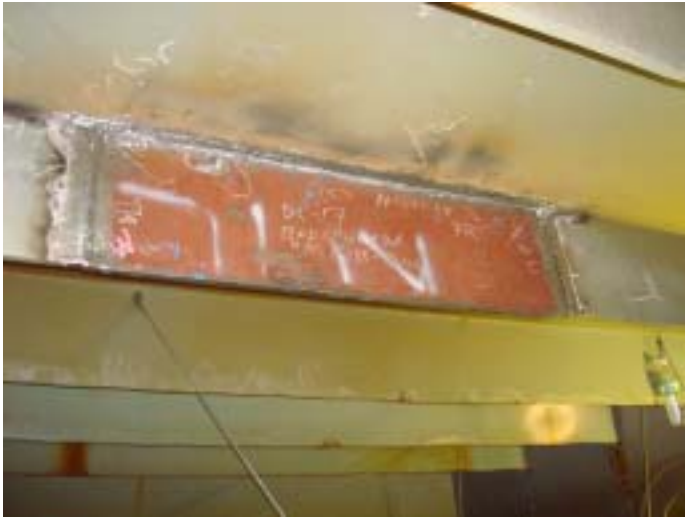
NO.6S DECK LONG.
