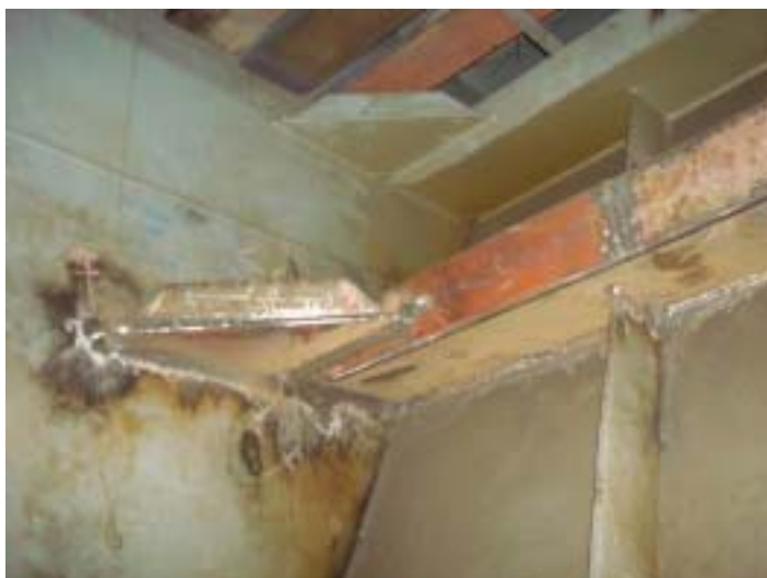
FOT Steel work
