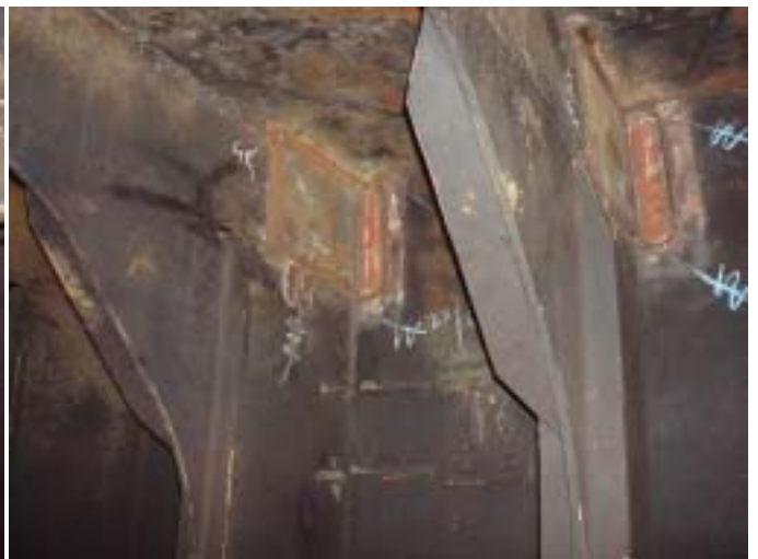
NO.3S steel work
