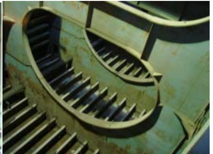
Close Tie on bottom in No.4S
