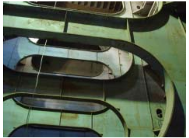
Close Tie in No.4S
