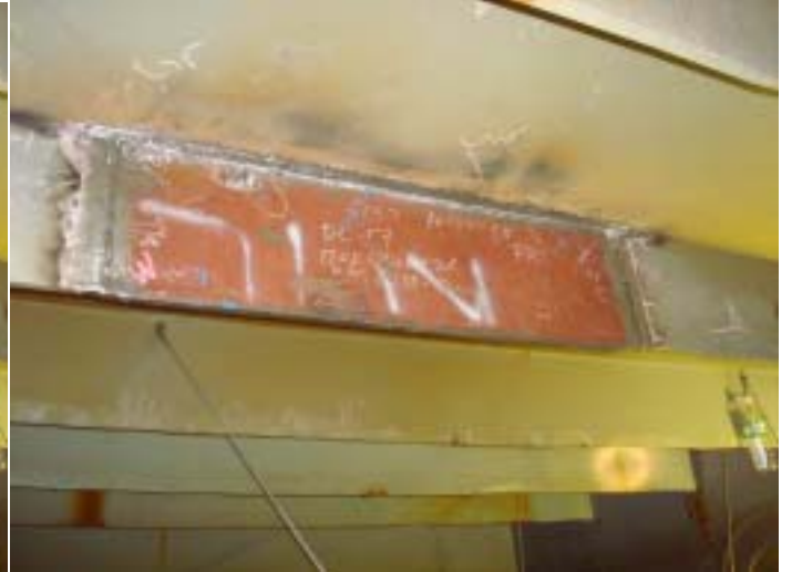
NO.6S DECK LONG
