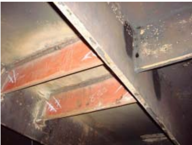
NO.5S steel work
