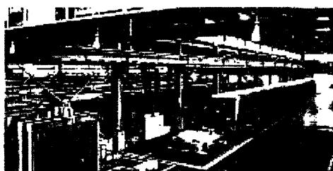
* 検修棟内観 Interior view of maintenance center
