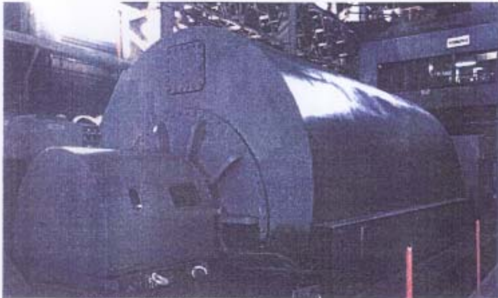
radial-vent-cooled turbine generator
